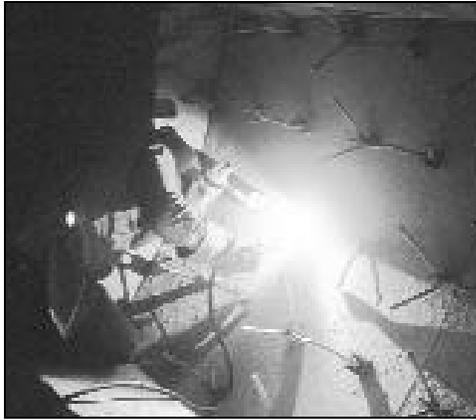
Figure 7 - Stick Welding Anchors
